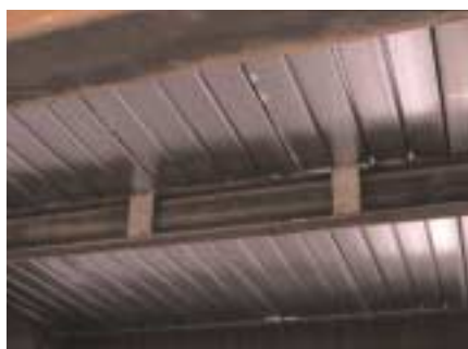
Noggings glued between steelwork flanges
