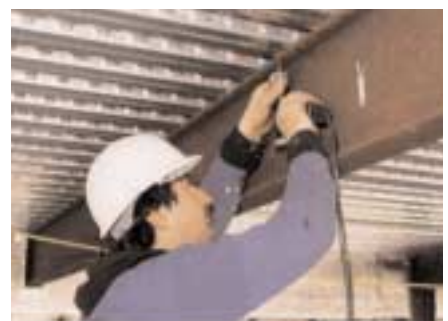
Fixing stud welded pins
